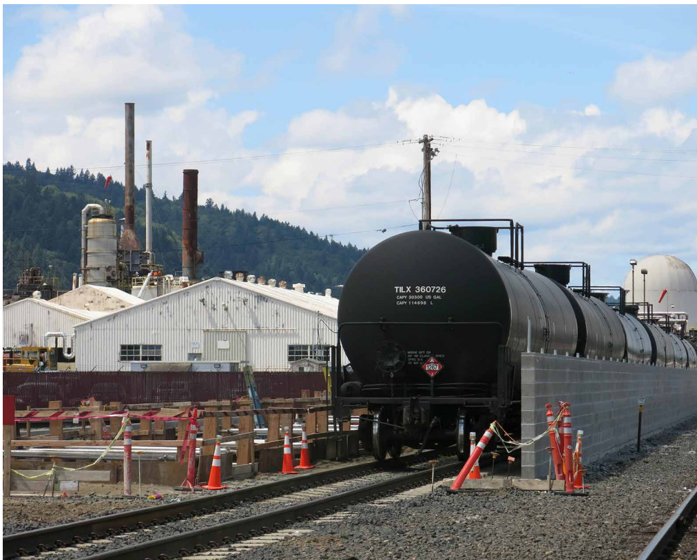
Zenith Energy terminal, Portland Oregon
