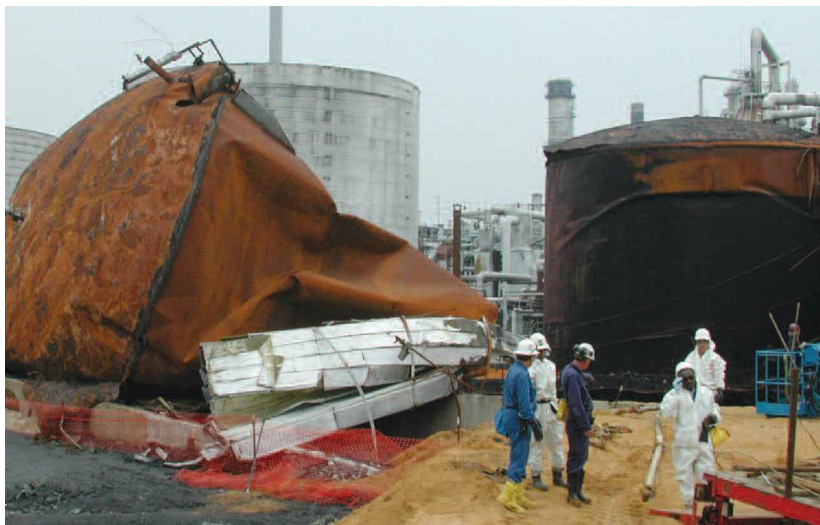
Aboveground storage tank explosion, Delaware, 2001.
